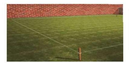
First you should mark all four corners of your building site using a wooden or metal stake. Run a string from corner to corner outlining the perimeter of your site.
